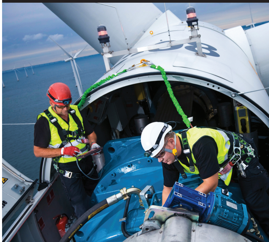
□ A crew accesses the inside of a turbine for maintenance.
