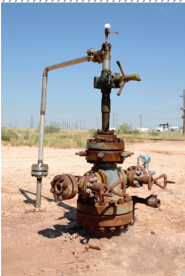
□ The CO 2 injection wellhead channels CO 2 and water about 3,000 feet down into the oil-bearing West Texas rock formations.
