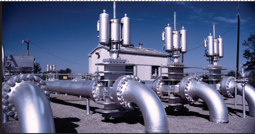
□ Gate valves with through-conduit and double block-and-bleed features along with fully protected seat faces work well for liquid pipeline applications.
