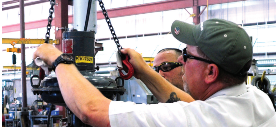
Control valve repair today involves skills and expertise that did not exist 20 years ago. VRC member companies have advanced their capabilities to meet the requirements of today's control valve repair.
