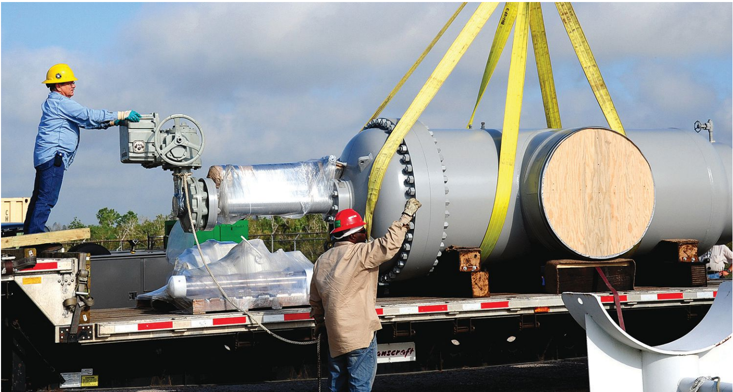
An NPS 36 pipeline-style parallel seat gate valve is unloaded at one of the U.S. Strategic Petroleum Reserve locations.
