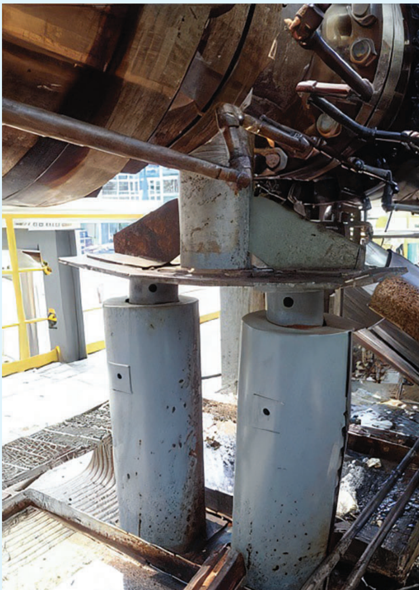
Figure 7: Piping supports are deformed from improper piping design failing to accommodate thermal expansion under large cyclic loads.
