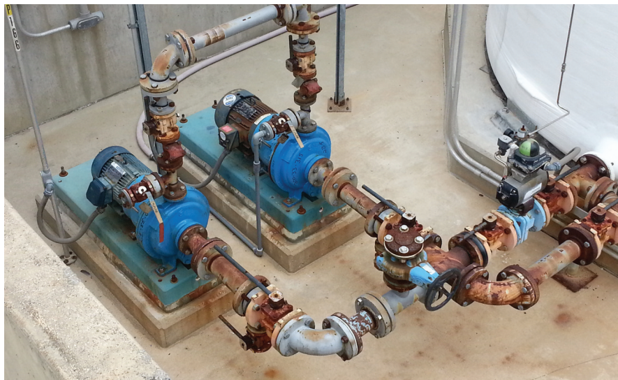
□ These pumps are used to unload bleach from tanks into a pulp and paper plant bleaching process. They use a seal-less design that eliminates failure that can result from crystallizing bleach.
