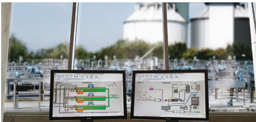
Remote control system
