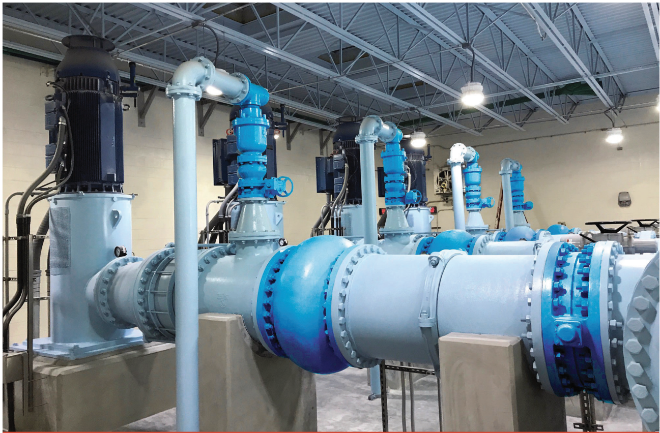
Pump station design with silent check valve installed five pipe diameter lengths from pump discharge.
