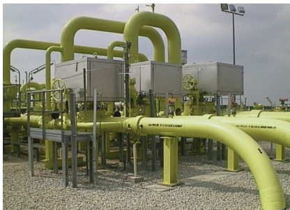
□ Fire-proofing systems provide a high level of protection for actuators and associated equipment in such critical areas as gas pipeline compressor stations.
