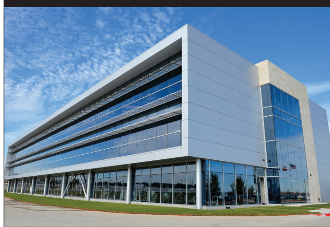
□ Emerson's new global regulator technologies headquarters building
