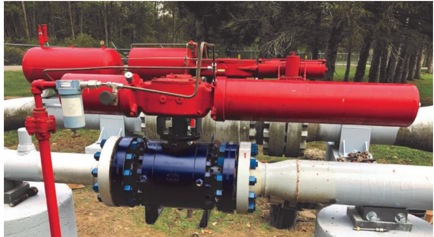
Trunnion mounted ball valve operated by a single acting spring return actuator.
