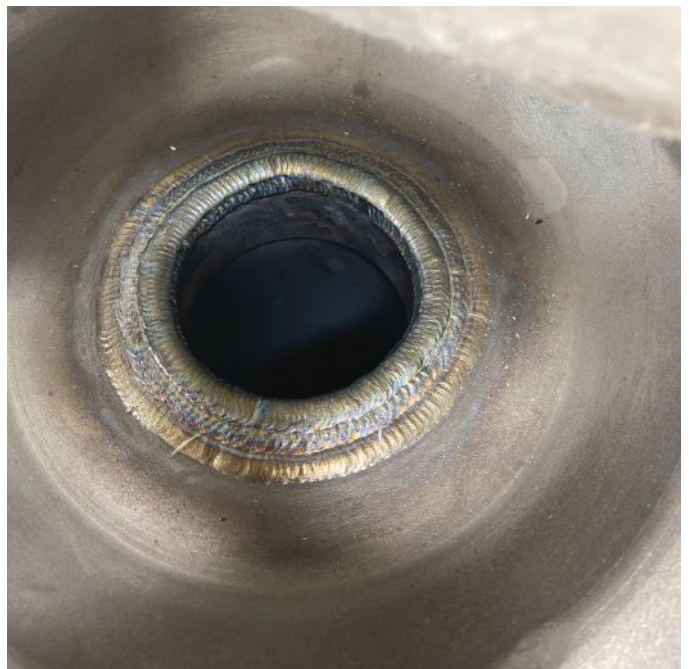
The same bonnet valve backseat post-repair.
