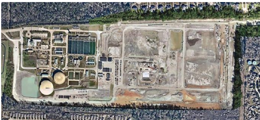
Aerial view of the existing plant (left) and area where expansion is currently underway.
