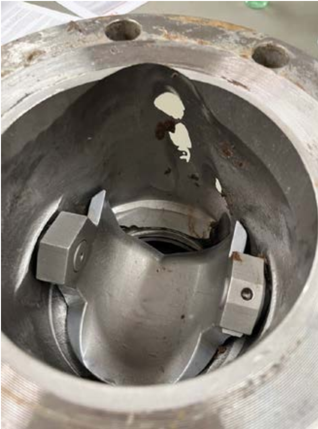
Internal photo of the same valve with holes highlighted, and erosion shown throughout on the ball of the valve.
